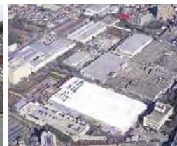
NSK Fujisawa Plant
