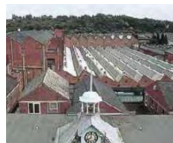
NSK Newark Plant
